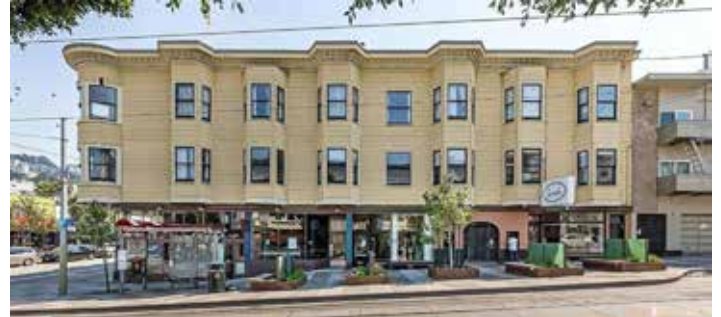
103 Carl Street recently underwent a "soft story" upgrade. No small task in a building this size.
