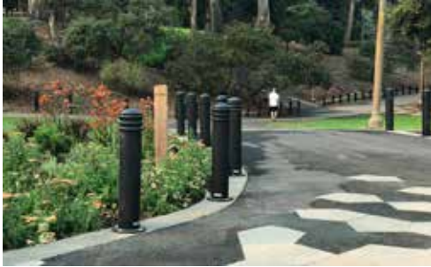
Planted areas are separated from the new path by bollards soon to be linked by chains.
