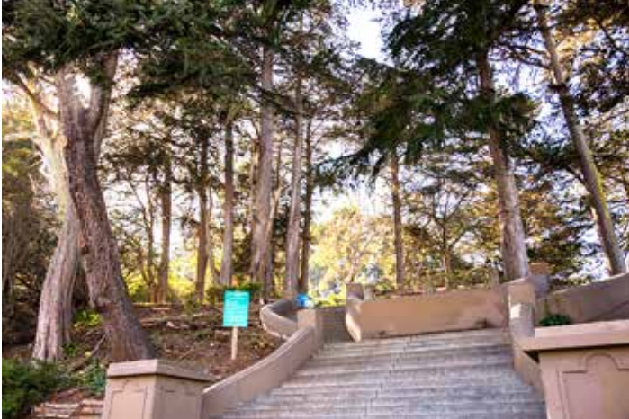
Park repairs will center on walkway safety issues.
