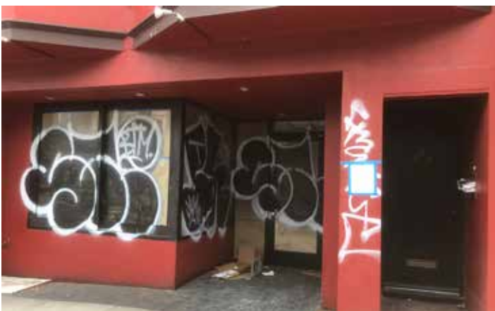
Reverie's long list of unheeded Building Inspection citations and needed upgrades are keeping this choice Cole Valley property empty. The Owner wanted $9,000 a month from prior tenant Roger Soudah, but who knows how much she will need after renovations? If Cole Hardware is the neighborhood's anchor, surely Reverie was its heart.
