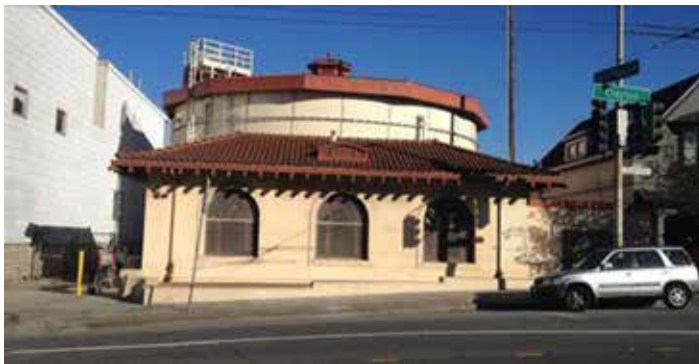
The 500,000 gallon water tank sits proudly on Clayton at 17th Street.
