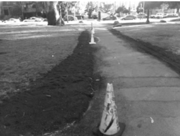
The Ashbury cross-over path from Fell to Oak is a work-in-progress.
