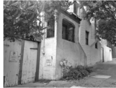
Existing building at 209 Grattan.
