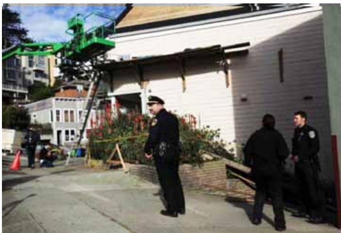
Makeshift scaffolding was nailed to the side of the building. When it collapsed, three workers were hospitalized.
