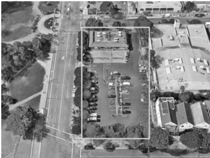
As part of the purchase agreement the existing McDonald's restaurant is scheduled for demolition leaving a vacant lot of 38,000 square feet.
