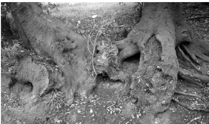
The slope on the south side of the entrance path is badly eroded.
