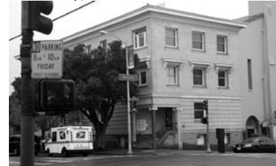
The wooden interior of the former Page Street Guesthouse will be replaced by concrete and steel.
