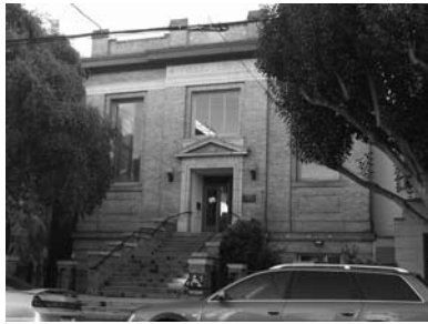
Users are leery that, once closed for renovation, the city's budget deficit will prevent the reopening of the Page St. library.
