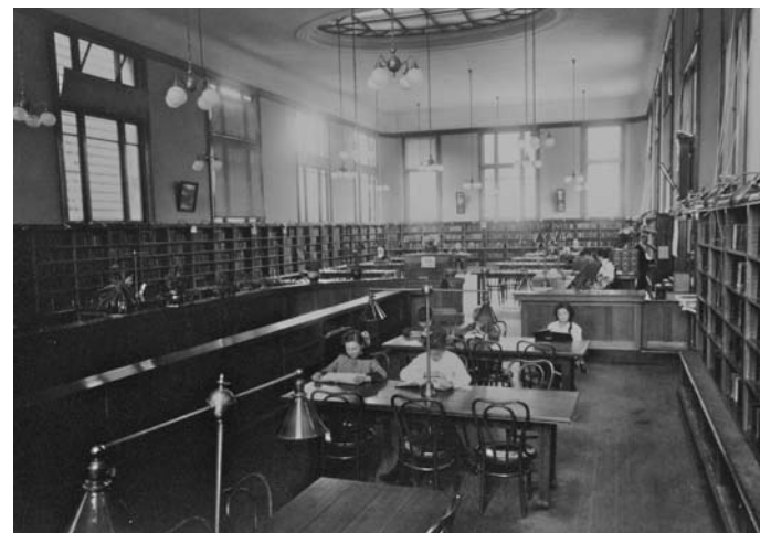
Shown here in 1916, the Park Branch is undergoing a year-long infrastructure upgrade requiring renovation or replacement of interior furnishings not covered by the Bond money.
