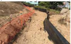
is finally underway. The new stairs will be box steps, constructed from Douglas Fir timber and compacted soil.
