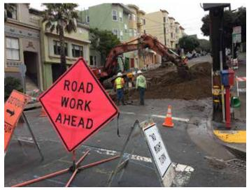
The Department of Public Works is methodically replacing the city's ageing sewer lines, some over one hundred years old. Neighbors watched as crews used excavators, front-end loaders and concrete mixers as part of a 20 year plan for infrastructure improvement.
