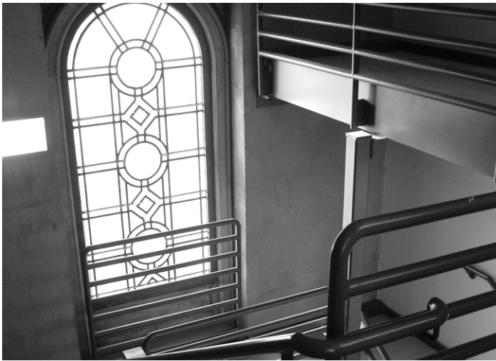
In this "building within a building," the historic exterior and modern interior meet only in the stairwell where an original window can be seen.
