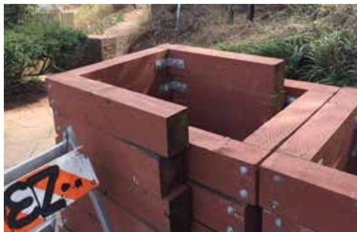
Old steps have been removed (top) and new "box" steps of douglas fir await installation.
