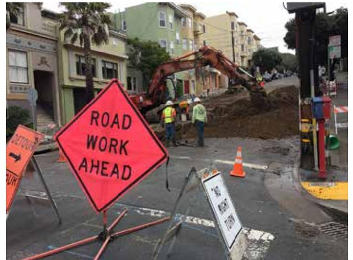
*The Department of Public Works is methodically replacing the city's ageing sewer lines, some over one hundred years old. Neighbors watched as crews used excavators, front-end loaders and concrete mixers as part of a 20 year plan for infrastructure improvement.*
